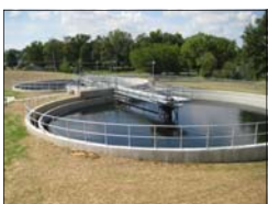
Oxidation ditch (top) and final clarifiers
